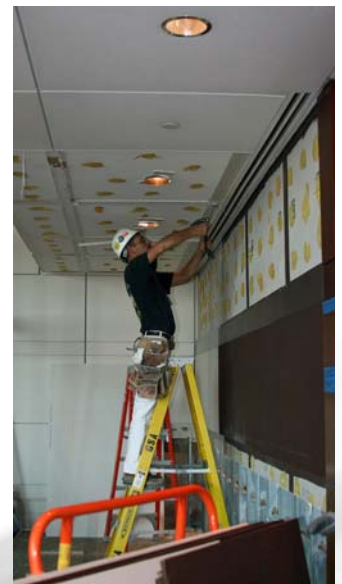
Flood repair work in Courtroom 13 South
